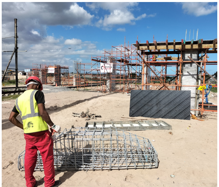
Construction of the pedestrian bridge is planned until December 2023.
