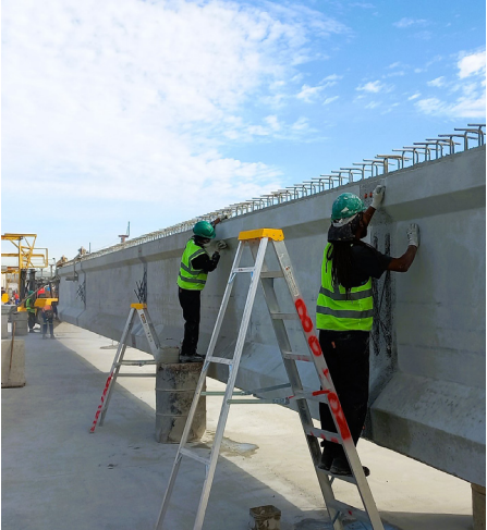
The enormous bridge beams have been cast off site by a local concrete company.
